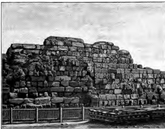
A SECTION OF THE SERVIAN WALL. (Present condition )
